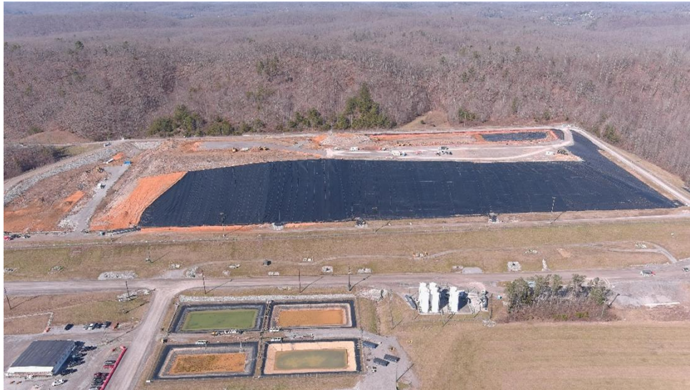
Environmental Management Waste Management Facility
