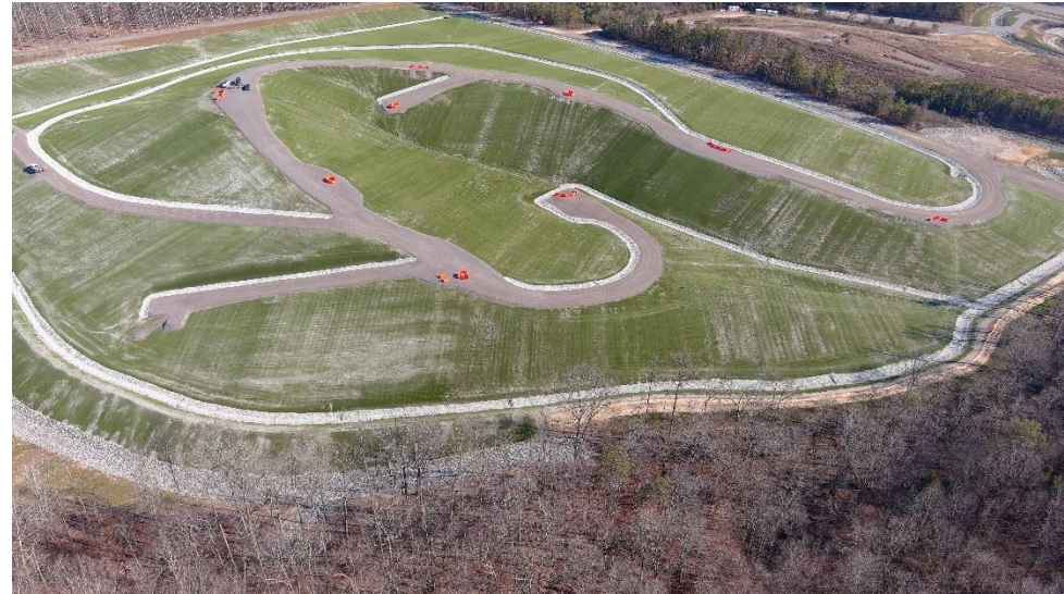
Environmental Management Disposal Facility
